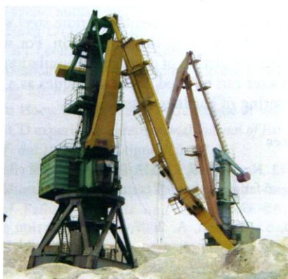
Fig. 1. Gantry crane accident
