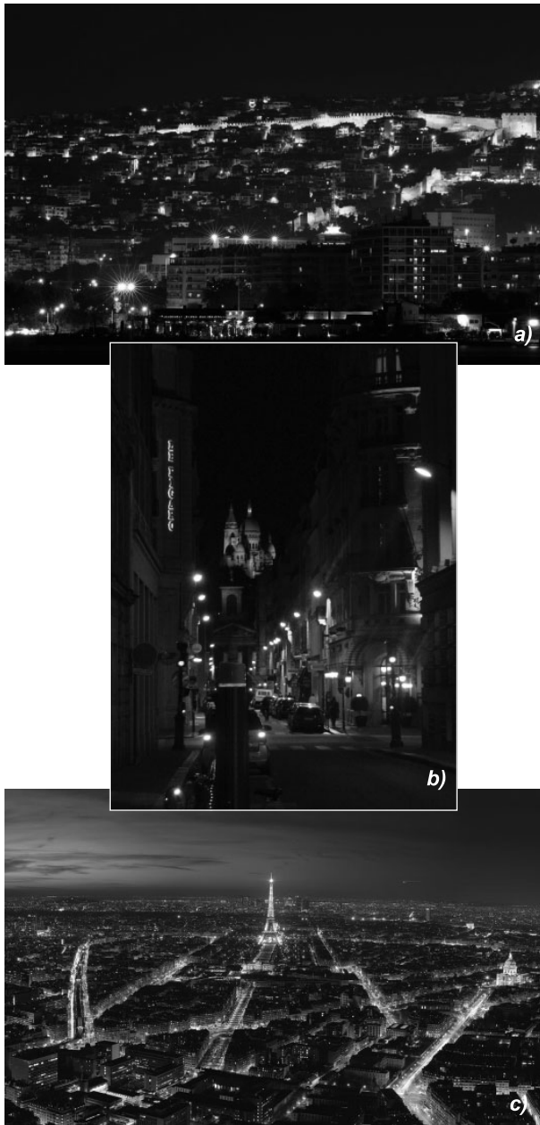
Fig. 5. Revealing architectural dominants by illumination. a) A fortress. Thessaloniki, Greece. Source: [8]; b) Basilique du Sacré Cœur. Paris, France. Photo: © 2012, M.Silkina; c) Tour d'Eiffel, Hotel des Invalides, Arc de Triomphe (light reference points) and a network of city streets (light frame). Paris, France. Source: [9]
