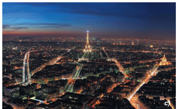
Fig. 5. Revealing architectural dominants by illumination. a) A fortress. Tessaloniki, Greece. Source: [8]; b) Basilique du Sacré Cœur. Paris, France. Photo: © 2012, M.Silkina; c) Tour d'Eiffel, Hotel des Invalides, Arc de Triomphe (light reference points) and a network of city streets (light frame). Paris, France. Source: [9]
