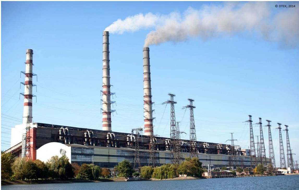
Fig. 1.1. View on the main hull of the Trypillya TPP
