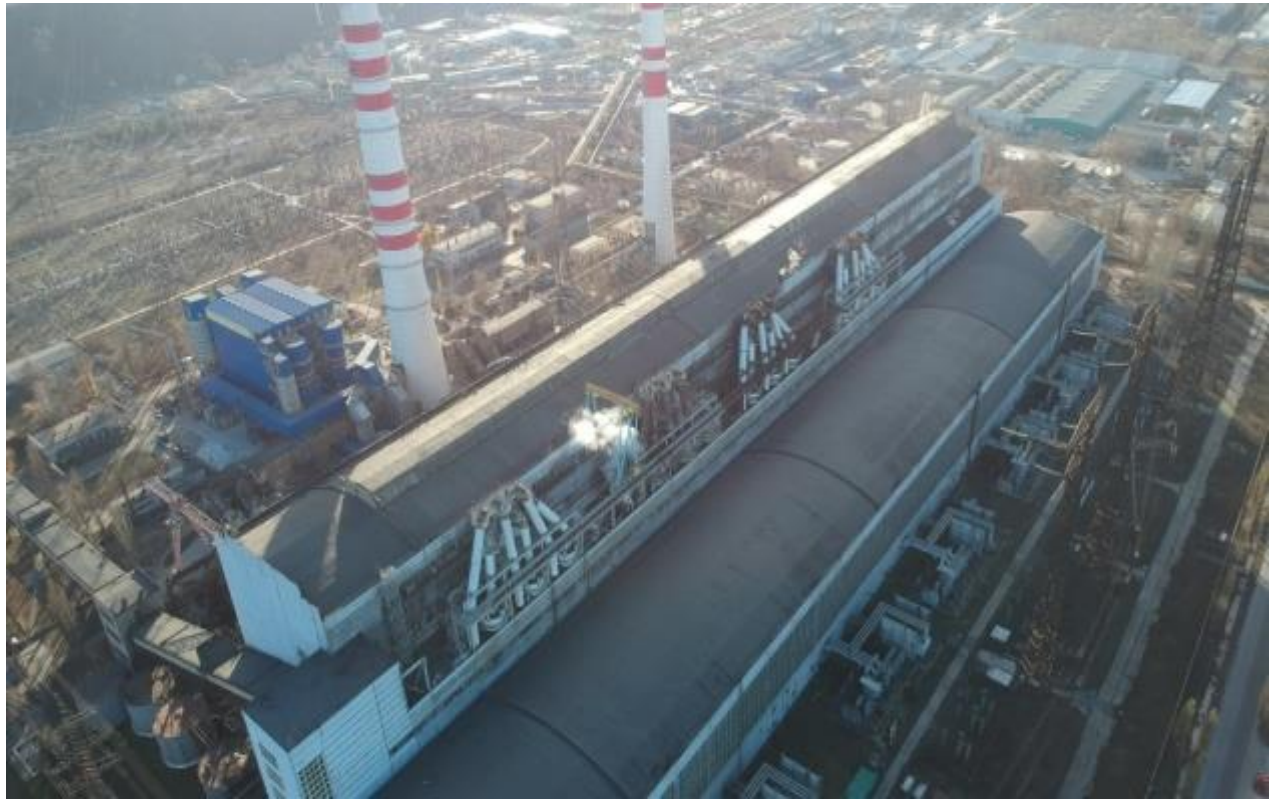
Fig. 1.3 As of 5 p.m., the occupiers fired a projectile into the coal depot of Trypillya TPP
