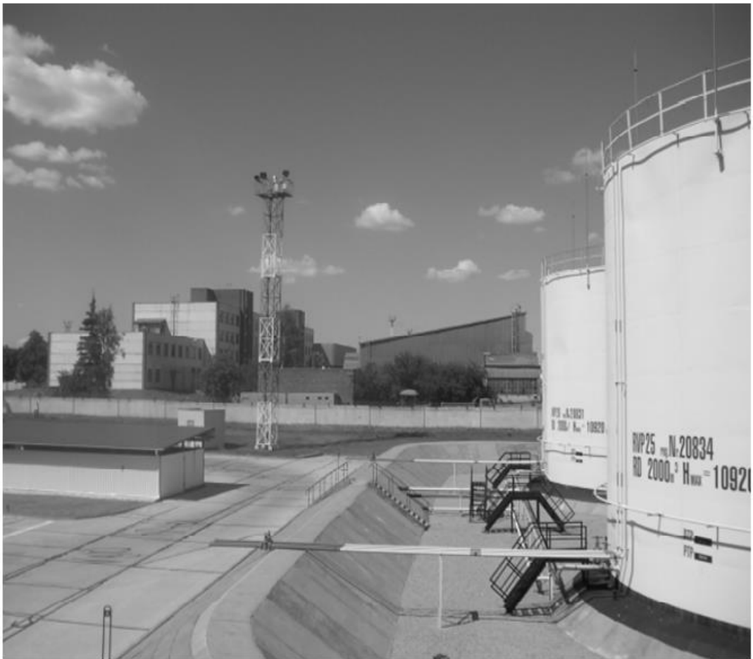
Fig. 26. Organization of solid concrete collapse of the fuel storage area
