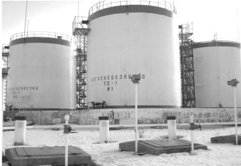
Fig. 20. Appearance of tanks at the fuel storage warehouse
