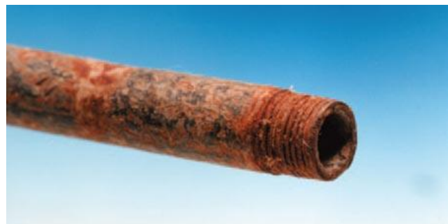
Figure 1.16 – Fretting-corrosion of the pipel.
