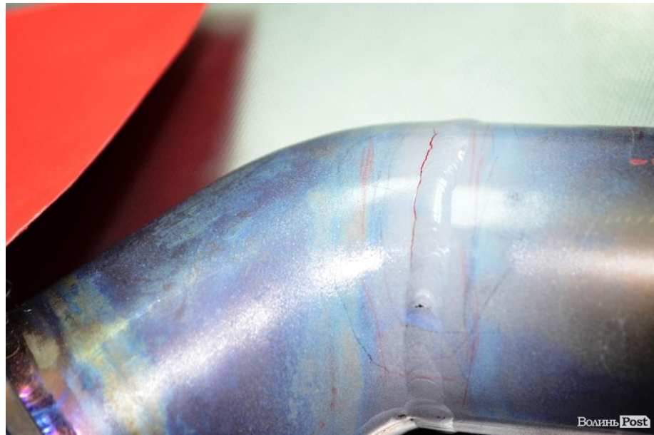
Figure 1.6 - Crack in pipelines
