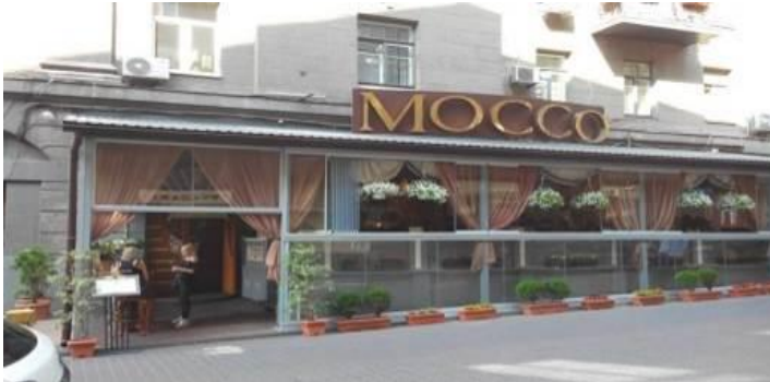
Fig.6. Entrance units of the “Mocco” restaurant
