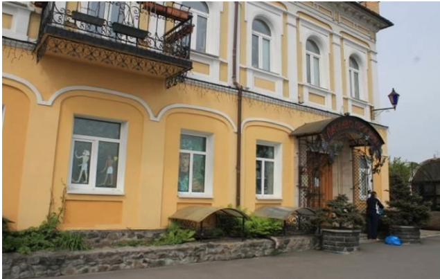
Fig.3. Entrance units of “Masandra” shop.
