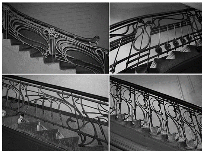
Fig. 8. Staircase fencing in the building № 26 at Chornovil Str. (1906); house № 5 at Vasylianky Str. (1911); house № 3 at Garkusha Str. (1912); building № 1 at Hrushevsky Str. (1910)
