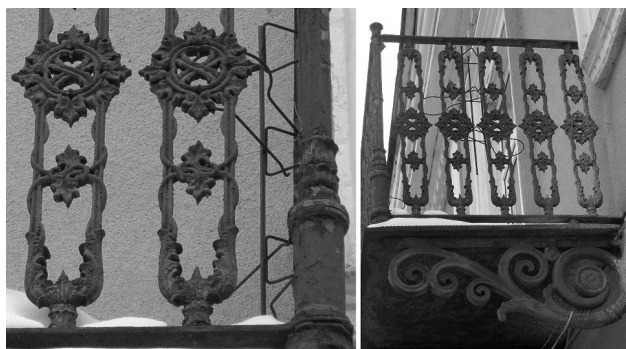
Fig. 3. Cast balcony fencing and brackets on the building situated at 1, Mazepa Str. – Vichevyi Square (dated 1827–1830)
