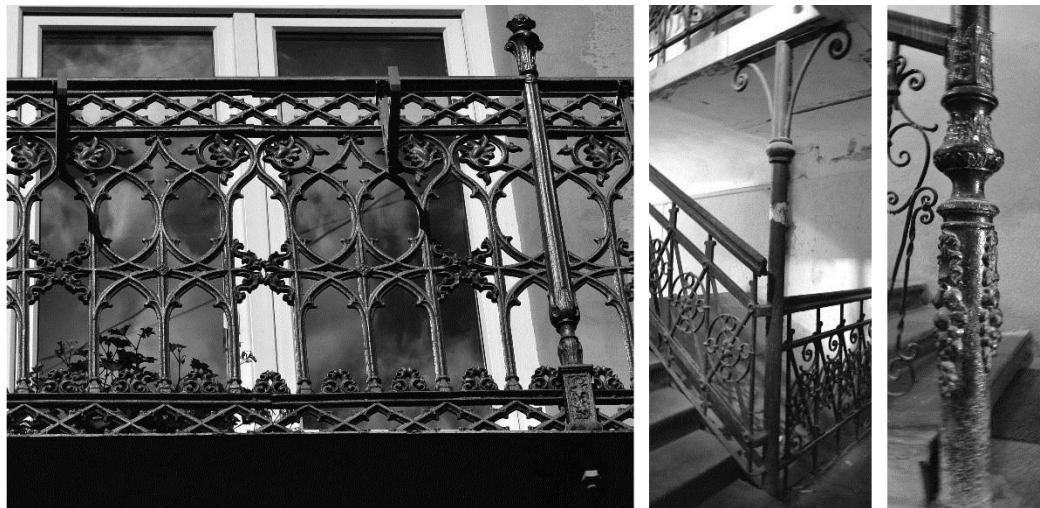
Fig. 5. Balcony fencing and brackets; staircase fencing; fragment of the decoration of staircase footing in the house №6 at Mazepa Str. (dated 1885)
