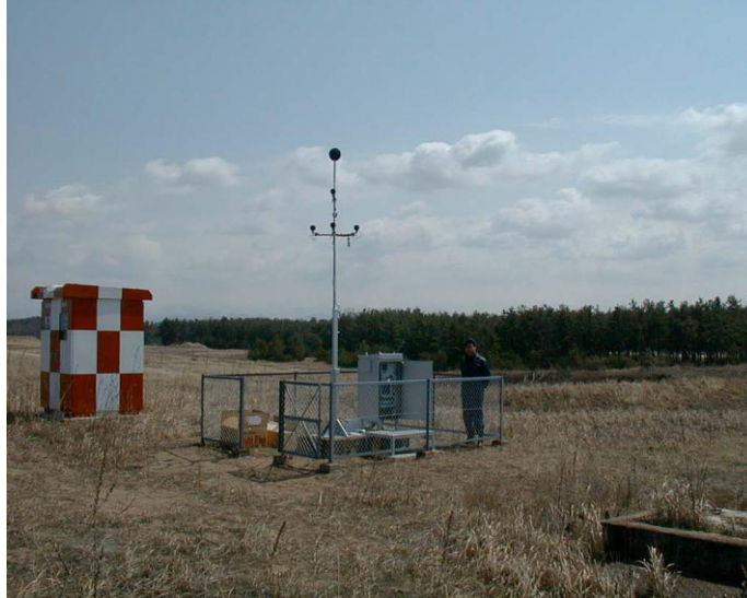
Figure 1. Noise monitoring terminal with 4 microphones system on a site [1]
