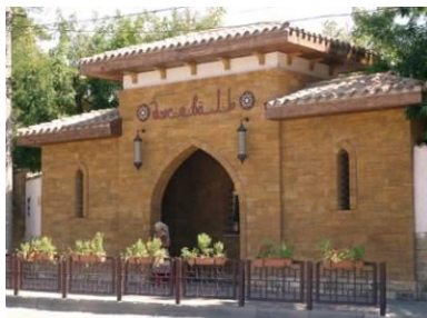
Fig.3 The entrance building of the restaurant “Dzewal”, 2009.
