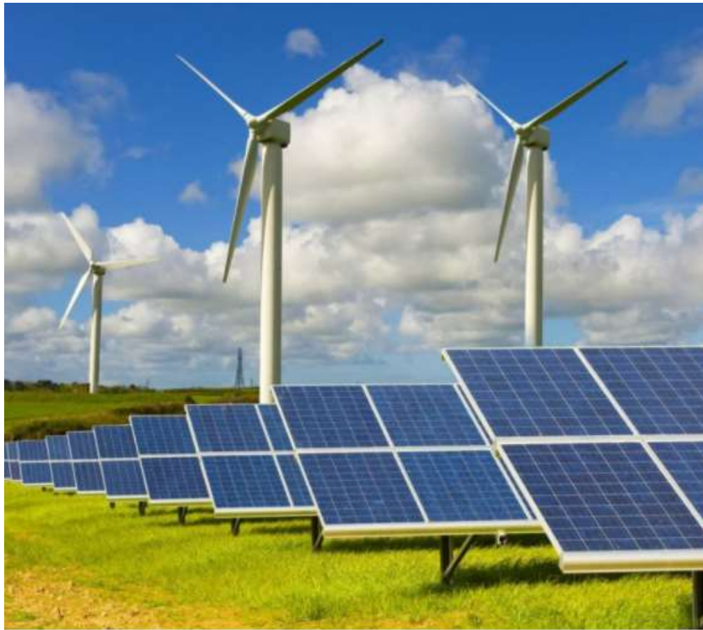
Fig.2.1 - Wind-solar hybrid plant
