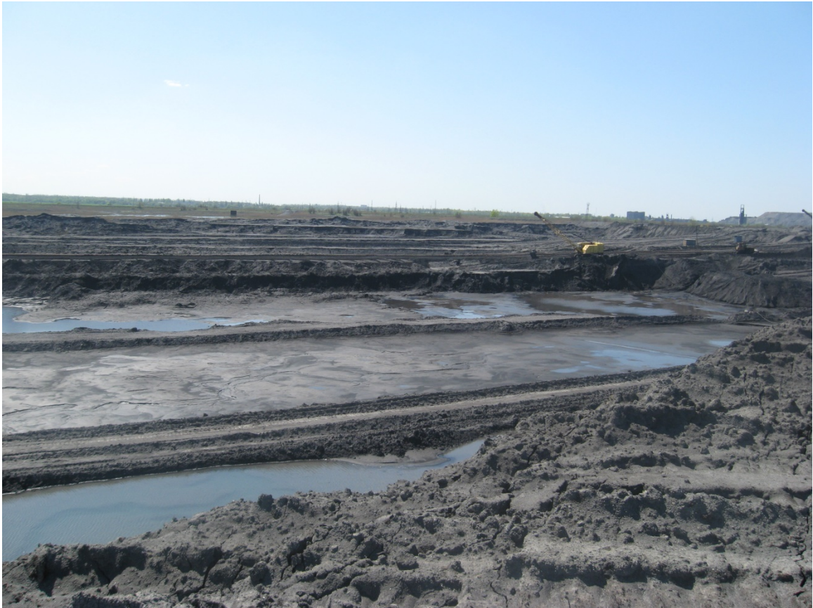
Fig. 2.2 Dry excavation in-process
