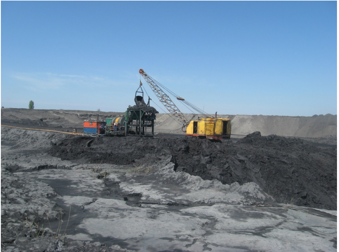
Fig 2.3 Construction of drainage canals and pouring of excavating ramps
