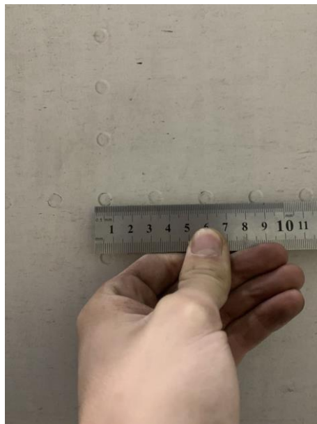
Fig. 2.3. – the distance between two riveted joints.
