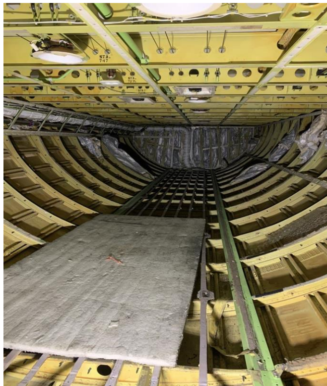
Fig. 1.11. – inspection of cargo compartment area.
