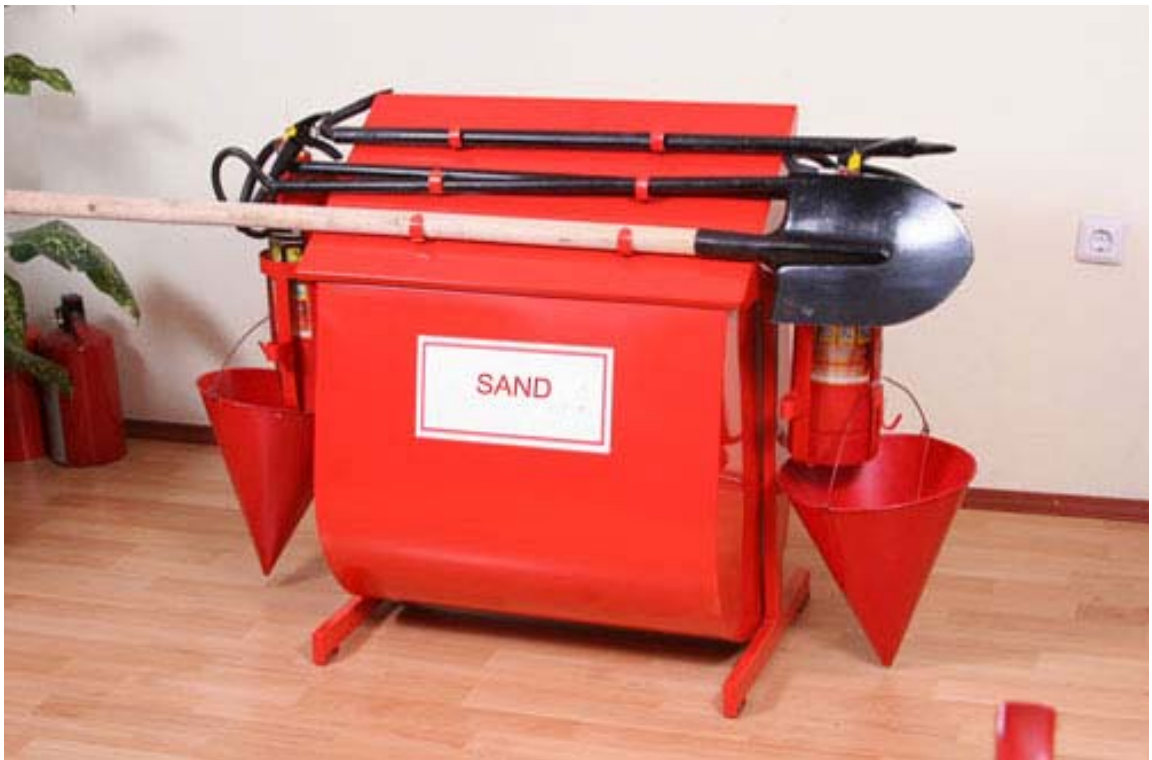
Fig. 4.11. Fire shield in the production room near the fire hazard of the workingearth.
